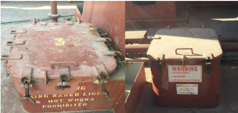
Figure 5 (upper left): No. 3 cargo hold access using the Australian ladder.
